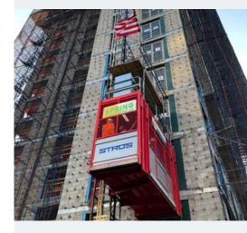
Among other applications, construction hoists are typically used on construction sites with high requirements for the transport of people and materials, in the construction of high-rise buildings and bridge pylons. STROS hoists are designed and manufactured for long life and reliability.
