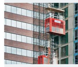
Among other applications, construction hoists are typically used on construction sites with high requirements for the transport of people and materials, in the construction of high-rise buildings and bridge pylons. Hoists are designed and manufactured for long life and reliability. The hoist can be in DUO design.
